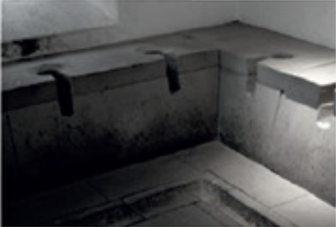
BATHHOUSE LATRINES There was also probably a bathhouse for the troops outside the fort. Its communal latrines had high-quality plumbing.
